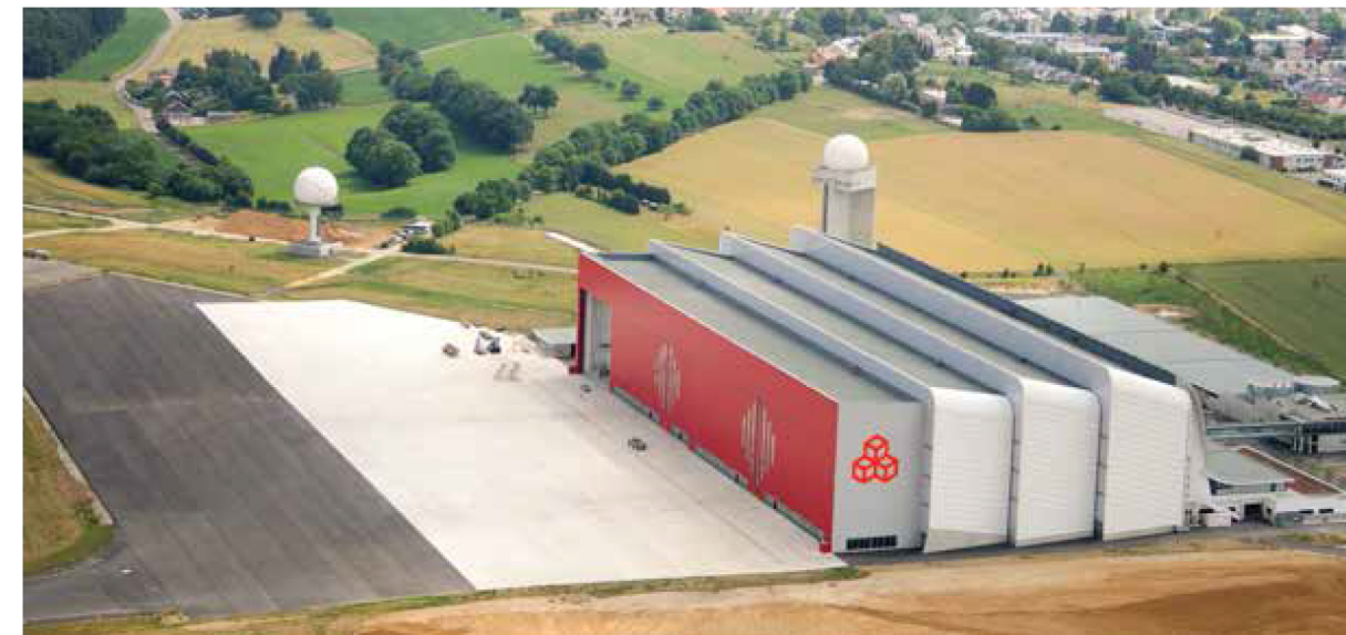
Cargolux maintenance hangar
